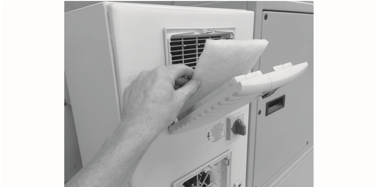
Fig. 39: Filter replacement in control cabinet
